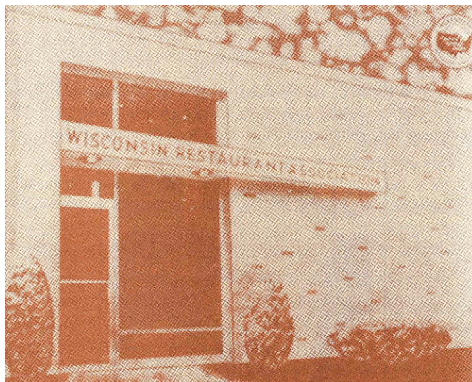
WRA office at 626 N. Van Buren Street in Milwaukee.
